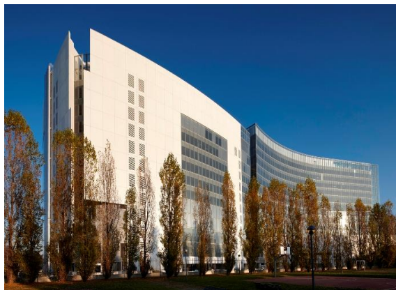
Vodafone Village (Mialn)
